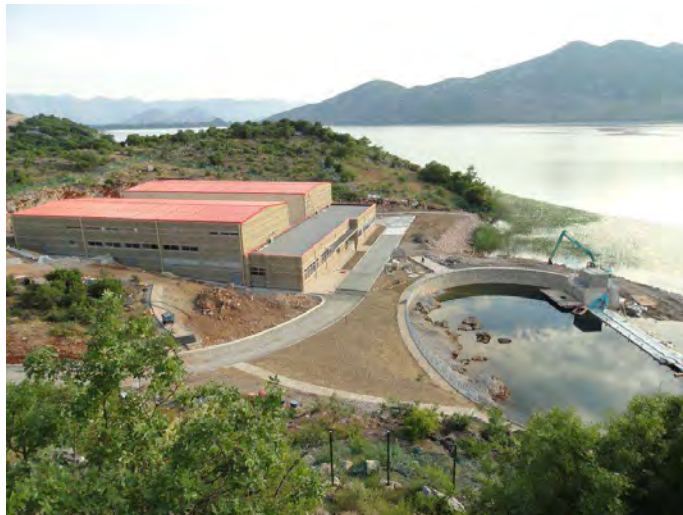
Fig. 6. Bolje Sestre spring (concrete built half circle on right side with small “dam” towards the Malo Blato lake on right side) view to the west with the pumping station building. “Dam” towards the lake has been built to prevent mixing/contamination of Bolje Sestre spring with lake water
